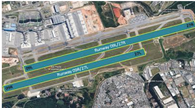
Fig-5: GRU runways. Source: Infraero, 2019
